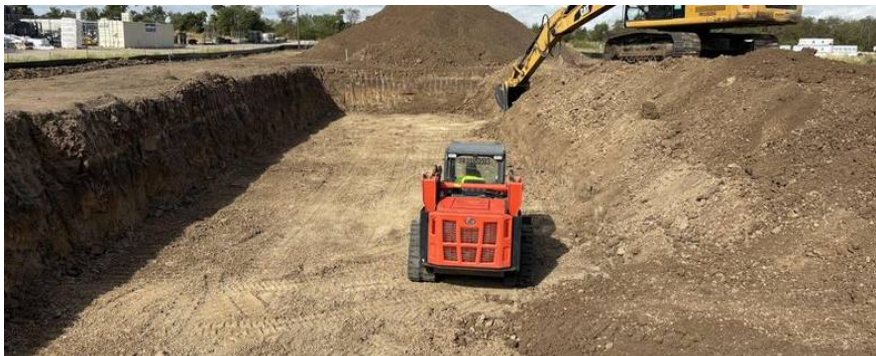
Excavator and track loader in a large commercial excavation (Circle H job photo)
